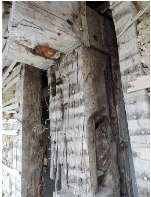
Fig.16 Le bûchage du poteau 102 © Rozenn Battais, Inrap
