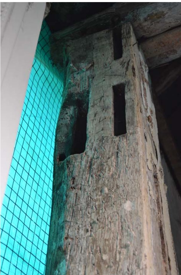
Fig.15 Les encoches hautes 316 © Elen Esnault, Inrap
