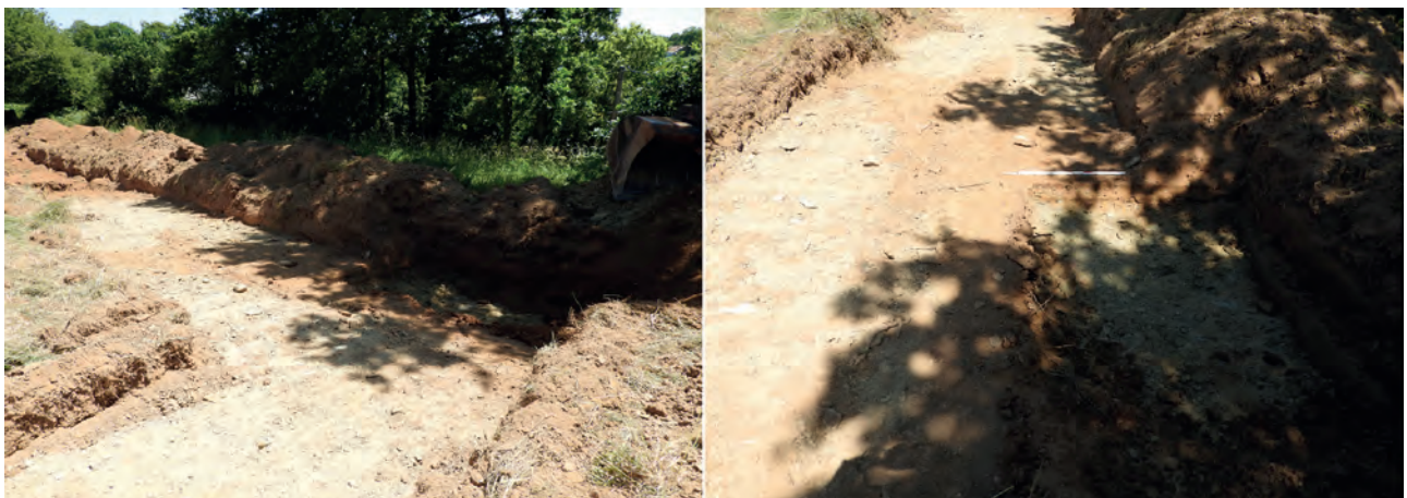
Fig. 5 La structure 4001. © Céline Baudoin
